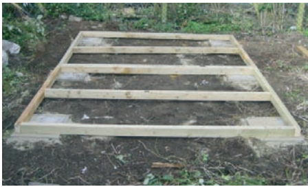
10x8 Raft on slabs laid on soil
