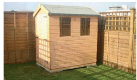
6x4 Apex shed on a raft laid on grass
