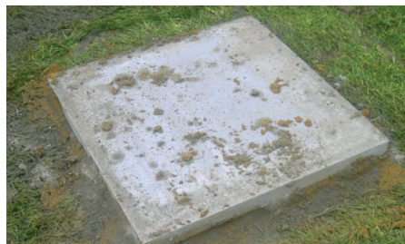
Slab laid on grass ready for a raft
